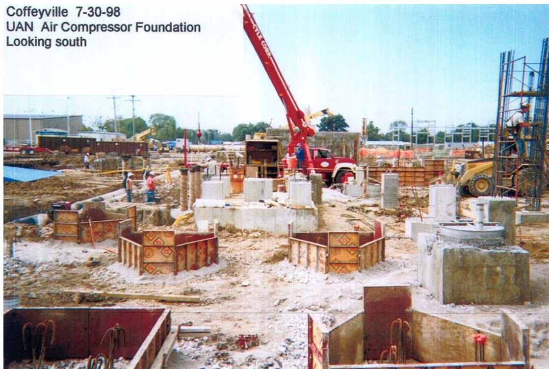
Fig. 6. R. 35, Ex. 508. Partially formed piers for the UAN Air Compressor.
