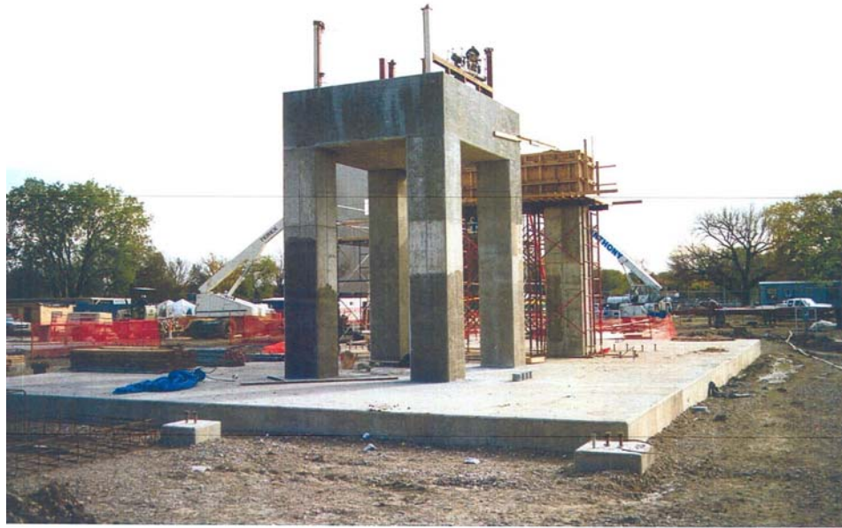
Fig. 5. R. 35, Ex. 503. Concrete foundation and supporting structure, under construction.
